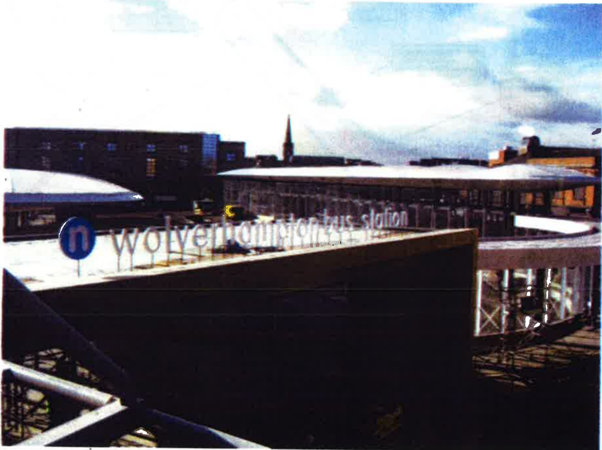
Work currently underway on the bus station
