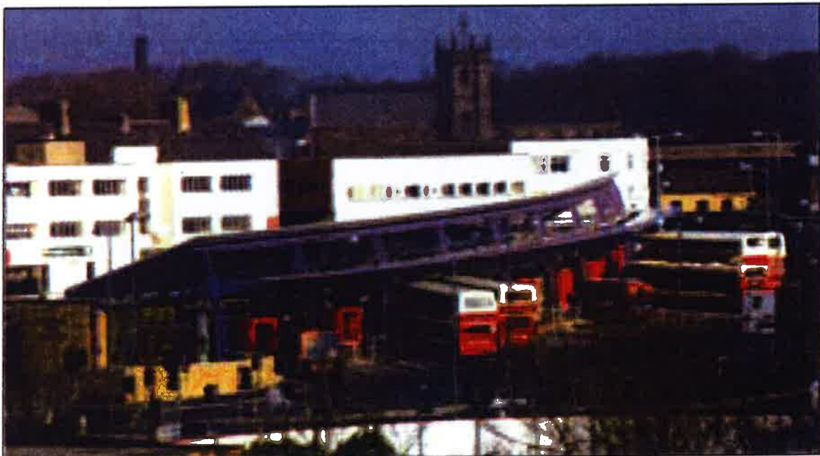
Figure 2.5: Burnley bus station bus circulating area
