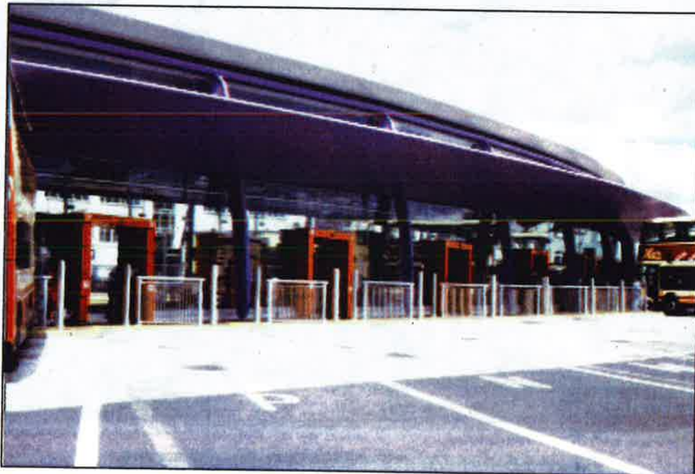
Figure 2.7: Burnley bus station bus departure bays
